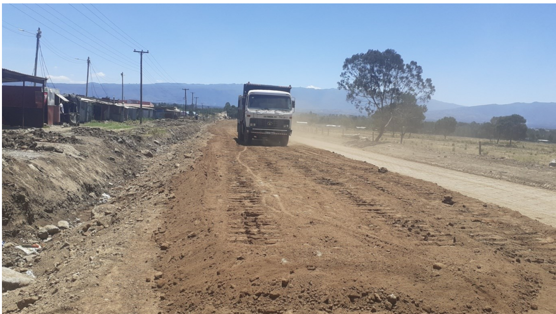
Figure 6-1: Ongoing road upgrade of D389
