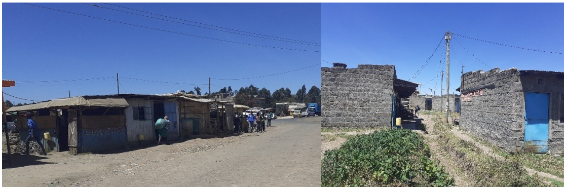
Figure 8-3: Type of wall and roofing material used
