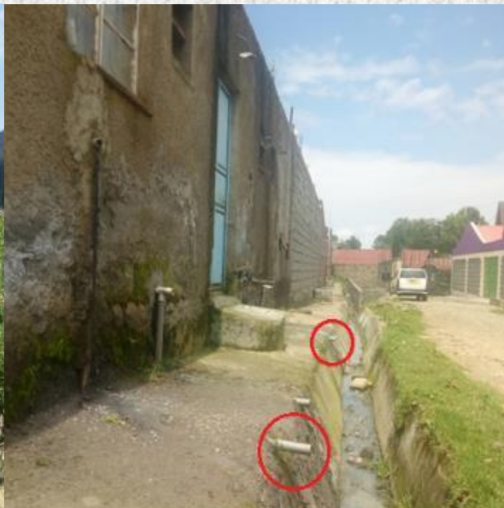
Discharge at Huruma Estate
